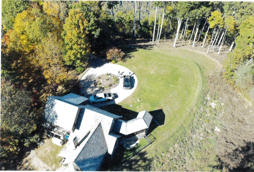
View 3 — Close aerial of existing structure and bench area adjacent to proposed site
